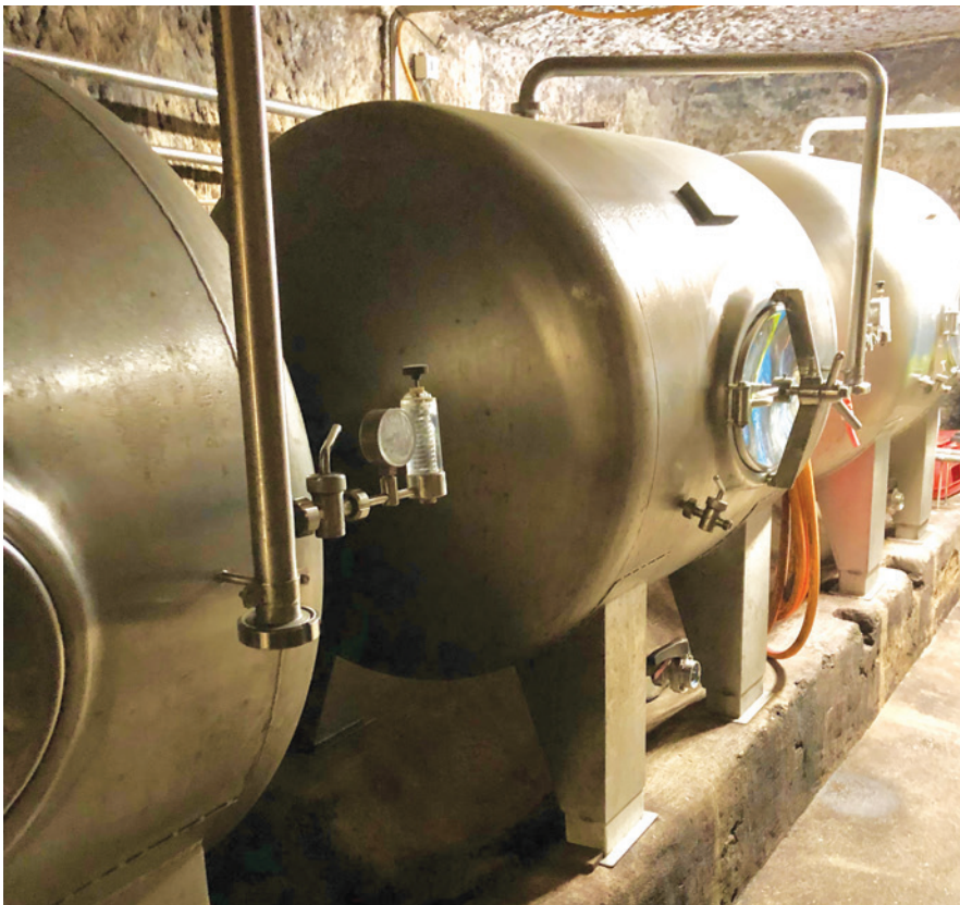
Horizontal fermenters inside the kellerbier cave of Schmausenkeller in Reundorf, Germany.
