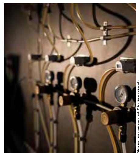
Bourdon gas pressure gauges allow brewers to measure the over pressure found inside sealed vessels such as kegs or unitanks.
