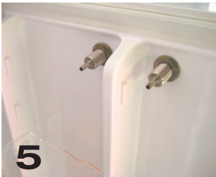
The shanks installed through the drilled holes. These can be sealed with caulk, if you feel that is necessary.
